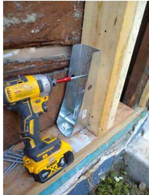
Hold-downs are installed at each end of all shear walls to resist uplift forces.
