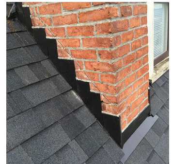
Fig. 1 Chimney stepped counter-flashing
