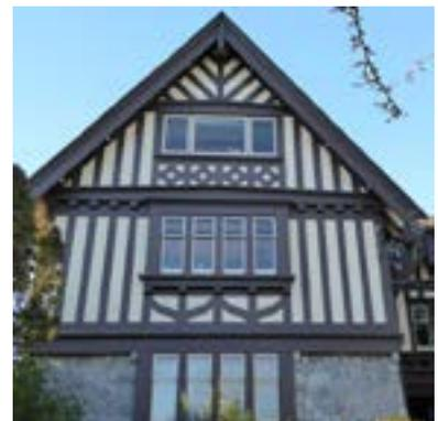
*Fig. 2 Wood half-timbering with stucco*
