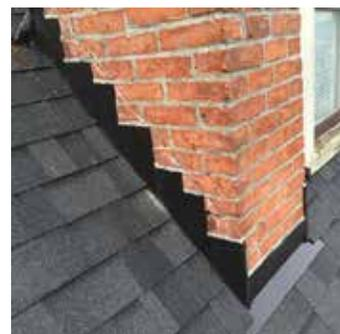
**Fig. 2** Chimney stepped counter-flashing
