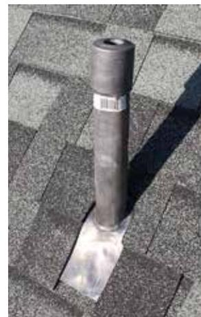
**Fig. 4** Lead plumbing stack flashing
