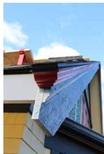
**Fig. 5** Gable edge drip flashing
