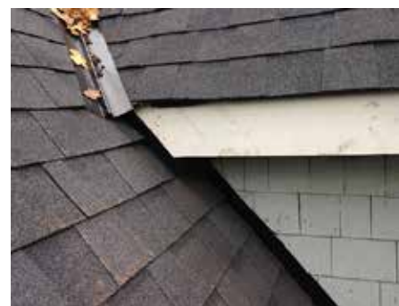
Fig. 1 Flashing is under siding at roof-wall intersections
