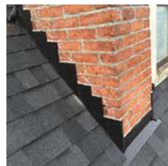
Fig. 2 Chimney stepped counter-flashing
