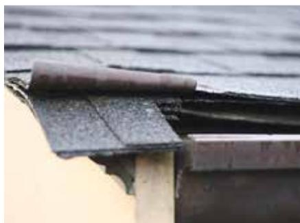
**Fig. 7** Metal rain diverter directs water into gutter
