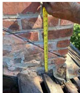
**Fig. 3** If previous counter-flashing was set into a diagonal groove cut into bricks, this must be repaired with colour-matched mortar.
