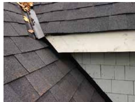
**Fig. 1** Flashing is under siding at roof-wall intersections
