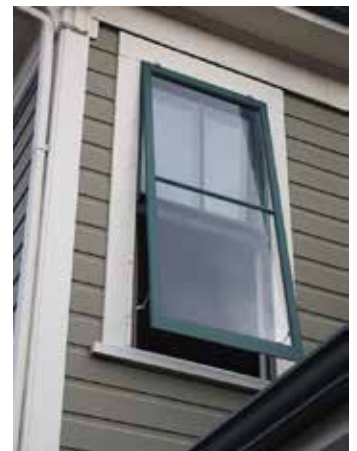
Fig. 2 Operable storm window attached with storm window hangers
