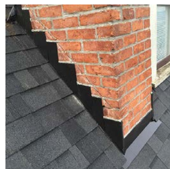
Fig. 1 Chimney stepped counter-flashing
