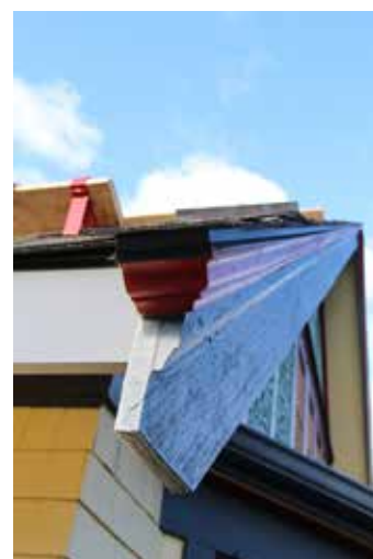
Fig. 5 Gable edge drip flashing
