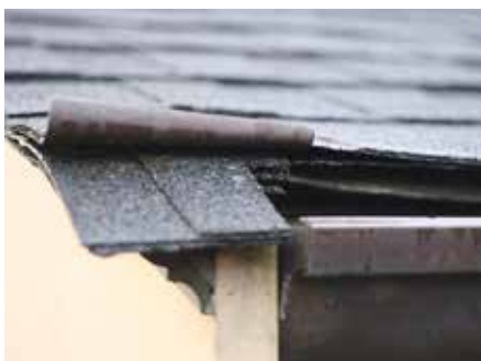
Fig. 7 Metal rain diverter directs water into gutter
