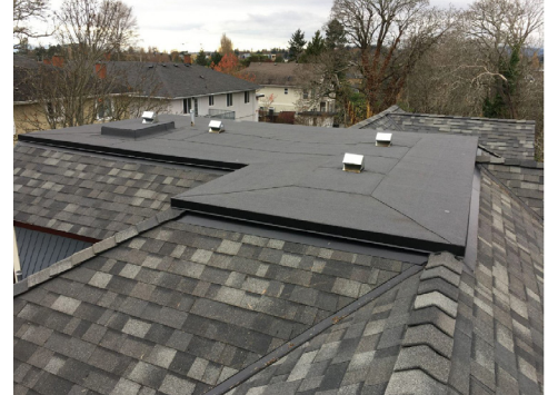
1116 Catherine St. roof replacement
