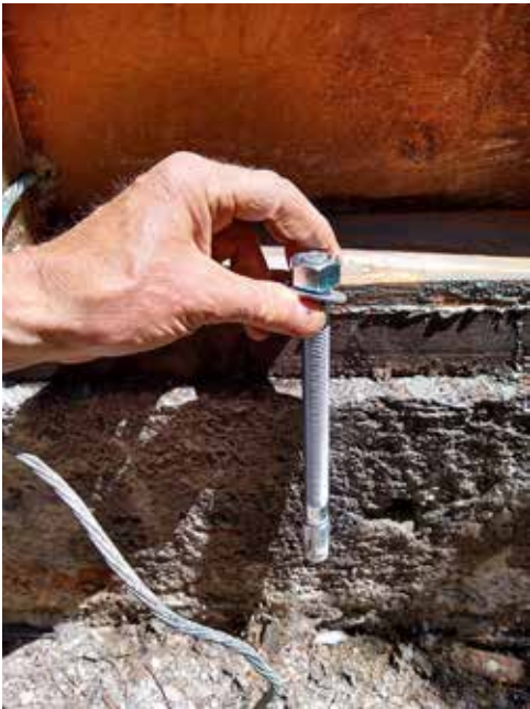
Anchor bolts strengthen the connection between the sill plate and foundation.
