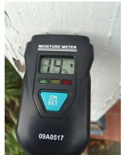
Fig. 1 Wood moisture content should not exceed 15% prior to painting.
