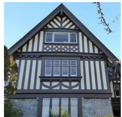
Fig. 2 Wood half-timbering with stucco
