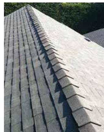
Fig. 8 High-profile ridge caps
