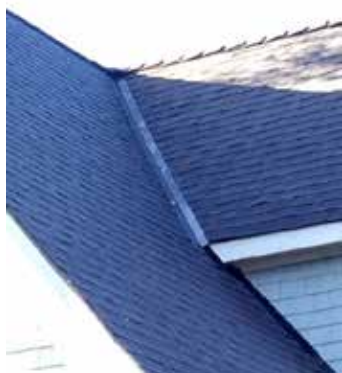
Fig. 6 Open valley shingling
