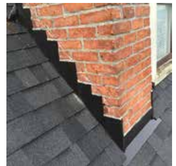
Fig. 2 Chimney stepped counter-flashing
