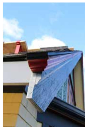
Fig. 5 Gable edge drip flashing
