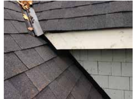
Fig. 1 Flashing is under siding at roof-wall intersections
