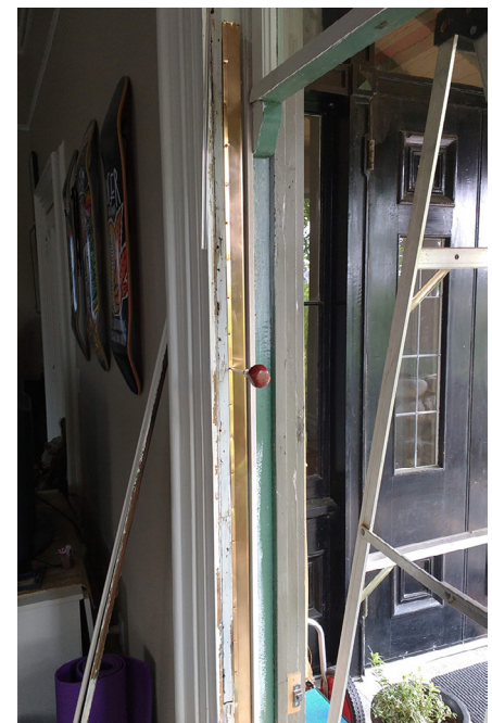
Fig. 2 Spring bronze weatherstripping installation in sash channel of double-hung window
