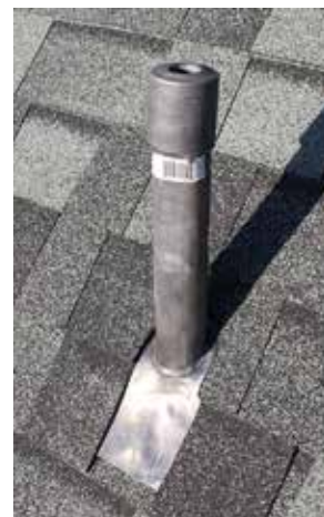
Fig. 4 Lead plumbing stack flashing
