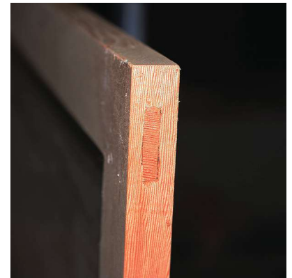
Fig. 1 Through-mortise and tenon joint
