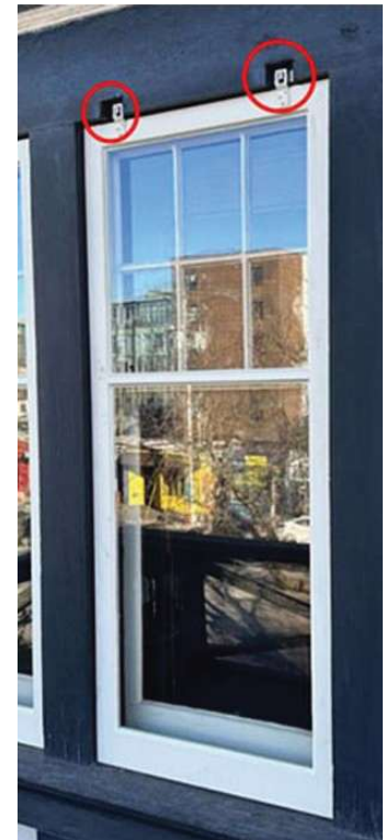
Fig. 4 Do not modify, cut or alter the building's character-defining elements when installing storm windows
