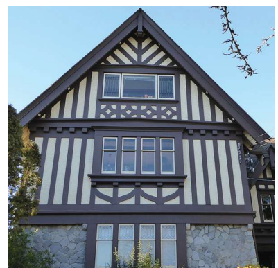
Fig. 2 Wood half-timbering with stucco
