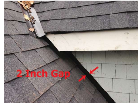
Fig. 1 Flashing is under siding at roof-wall intersections
