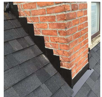
Fig. 2 Chimney stepped counter-flashing
