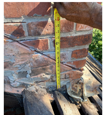
Fig. 3 If previous counter-flashing was set into a diagonal groove cut into bricks, this must be repaired with colour-matched mortar.
