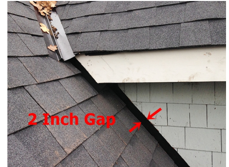
Fig. 1 Flashing is under siding at roof-wall intersections
