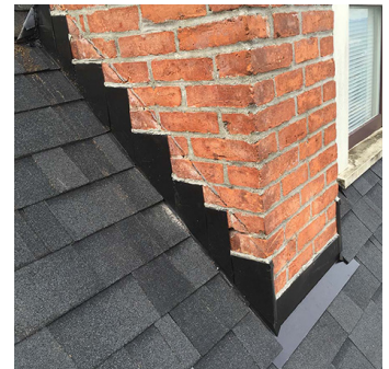
Fig. 2 Chimney stepped counter-flashing
