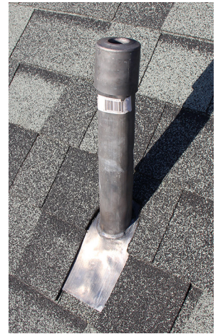
Fig. 4 Lead plumbing stack flashing
