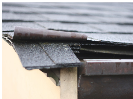
Fig. 7 Metal rain diverter directs water into gutter
