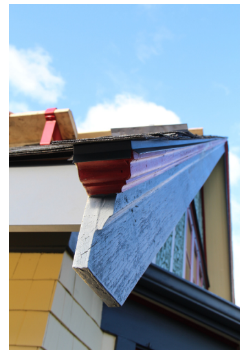
Fig. 5 Gable edge drip flashing
